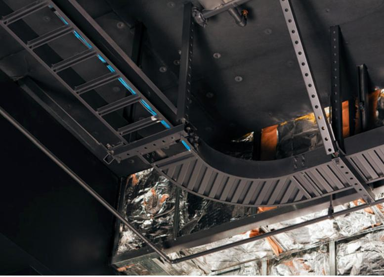
An extensive infrastructure of cable trays and conduit travel above and below the stage and audience area in order to accommodate current and future applications and technologies.
