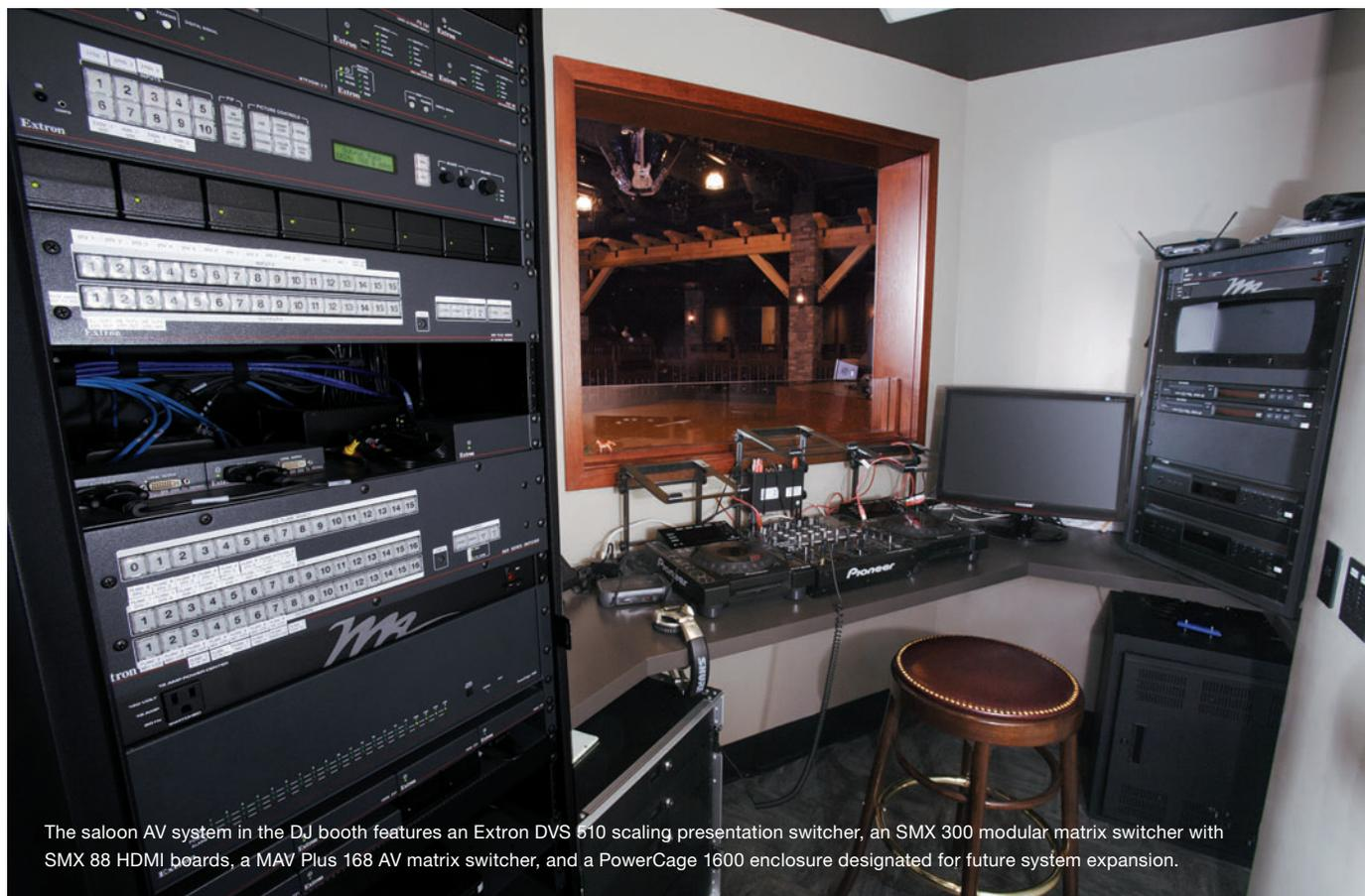
The saloon AV system in the DJ booth features an Extron DVS 510 scaling presentation switcher, an SMX 300 modular matrix switcher with SMX 88 HDMI boards, a MAV Plus 168 AV matrix switcher, and a PowerCage 1600 enclosure designated for future system expansion.
